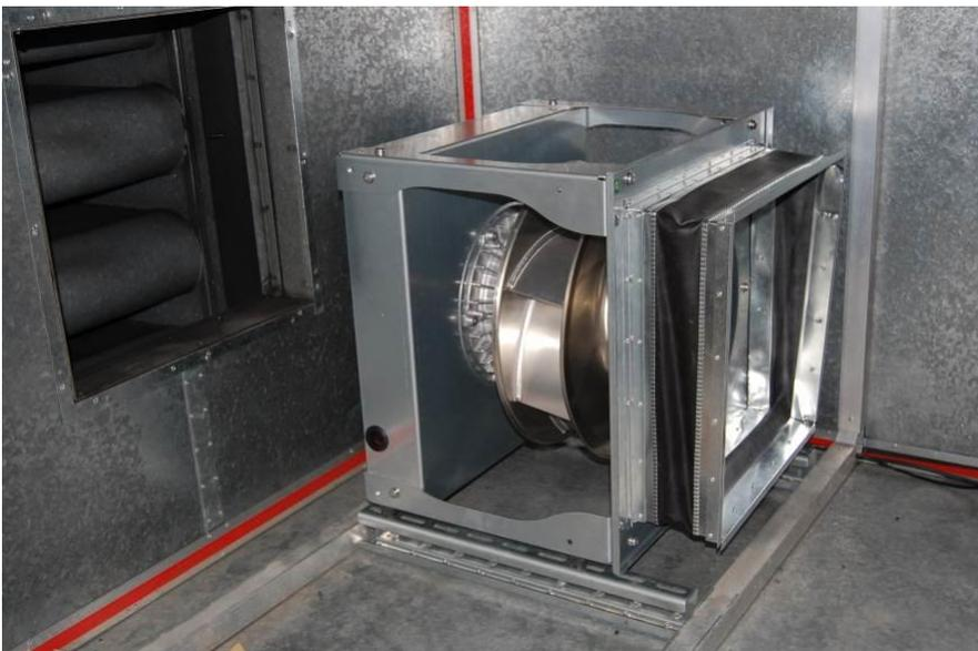
Fig 2: The RadiPac fans from ebm-papst in the air handling unit.
