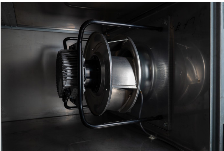
Image 2: Efficient RadiPac EC fans from ebm-papst replace the old AC technology.
