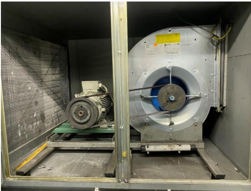
Fig. 2: The old belt-driven fans used too much electricity and the air performance was not sufficient for newer hospital extensions.
