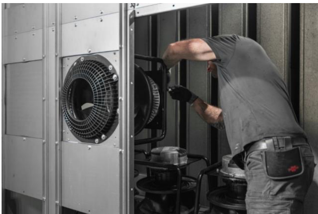
Fig. 2a: A FanGrid with several fans running in parallel provides a high level of operational reliability.
