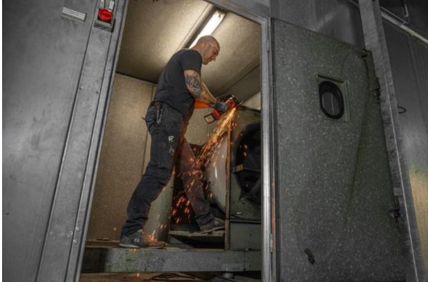
Fig. 1: The old fans were too large to be removed from the plant room in one piece and had to be dismantled into individual parts beforehand.
