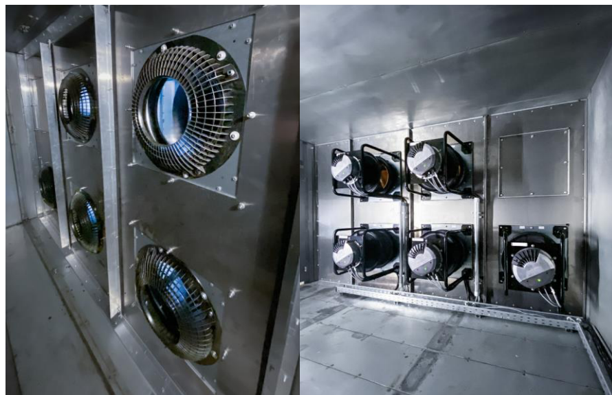
Figs. 2 and 3: The FanGrid was designed to make it easy to install another fan at any time. The opening for this is covered by a flap. The five RadiPac C EC fans ensure the necessary system redundancy.
