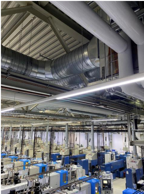
Fig. 1: In Hall 2, the exhaust air from the machinery is extracted via the ventilation system. This places special demands on its operational reliability.
