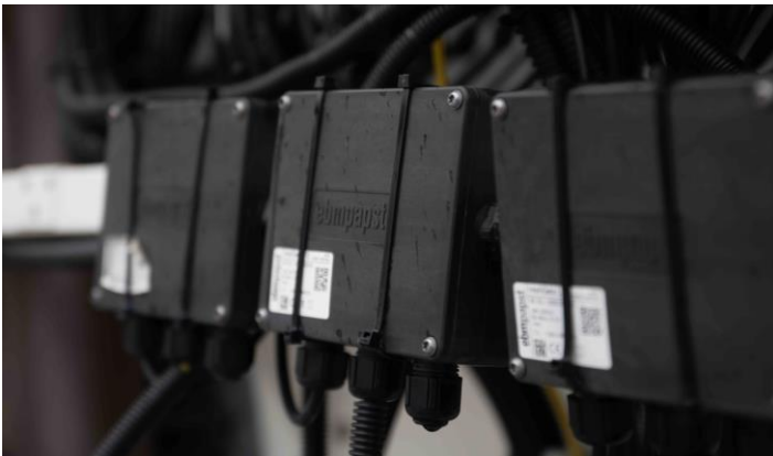
Picture 2: All the data from the new sensors converges at the gateways and is uploaded to the epCloud.
