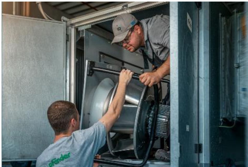
Figure 2: In many systems, EC fans were replaced with the latest generation of EC fans.
