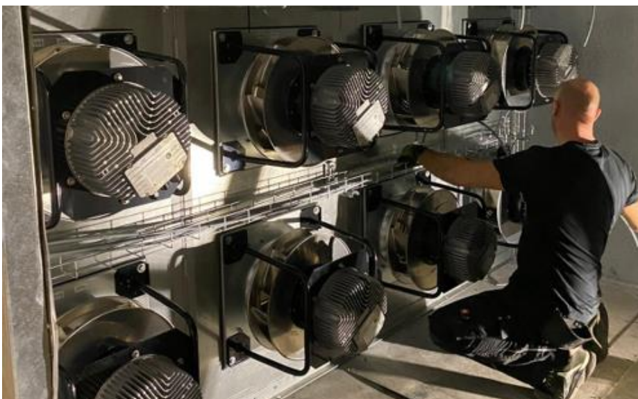
Caption: The Zeithaus automobile museum houses vehicle after vehicle. After a retrofit, the new ventilation system follows suit: one FanGrid houses RadiPac after RadiPac and saves 25 % in energy. (Photo: ebm-papst)
