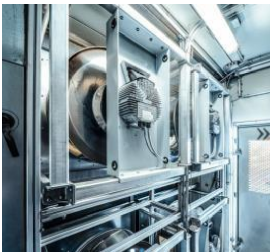
Fig. 2: The new ventilation system with a total of 16 RadiPac EC fans ensures that the dairy products remain fresh at a constant five degrees Celsius.
