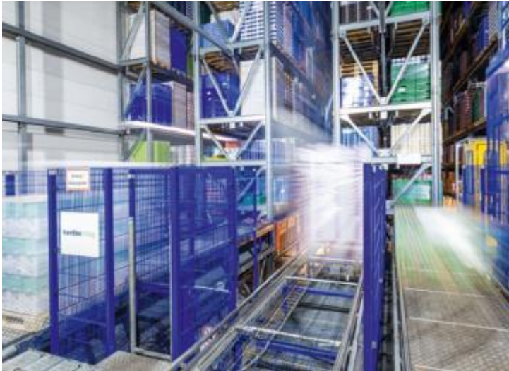
Fig. 1: The operational reliability of the ventilation system is a central aspect for the high-bay warehouse of Elsdorfer Molkerei with pallets full of perishable goods.
