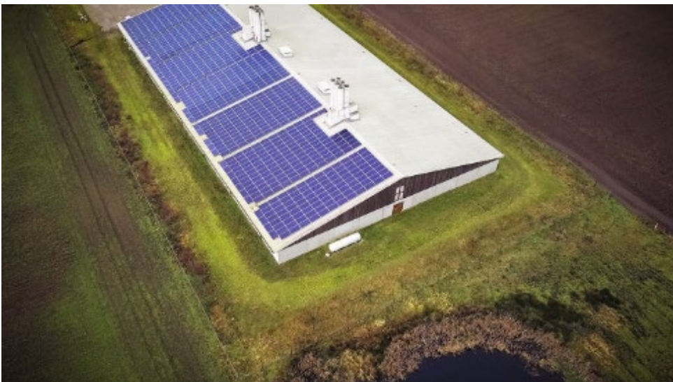
Fig. 3: The pig barn at the Momeyer's farm near Celle was equipped with new ebm-papst fans for ventilation and now saves over 50% of the electricity costs.
