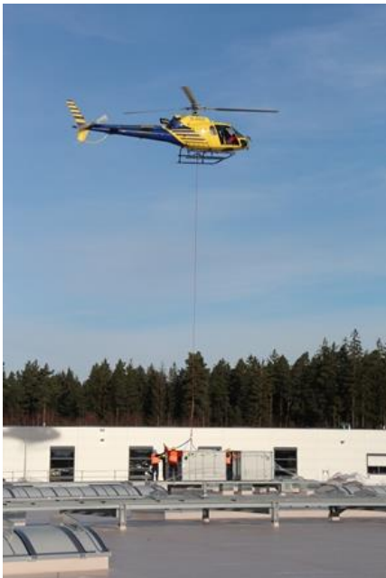
Fig. 1: Delivery via helicopter
