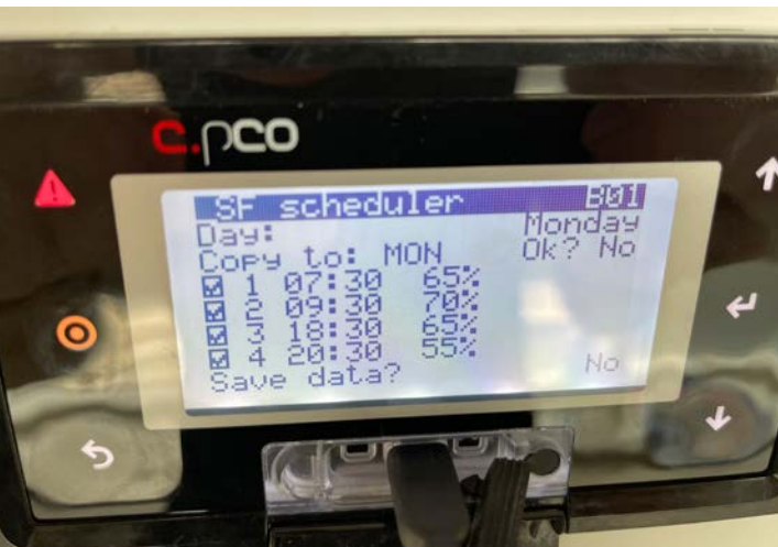
FIGURE 4: The demand-based control system regulates the air volume flow depending on the time.
