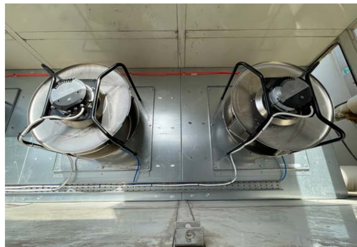
FIGURE 3: In a FanGrid, the RadiPacs are installed next to or above one another and operated in parallel. This ensures particularly high operational reliability.
