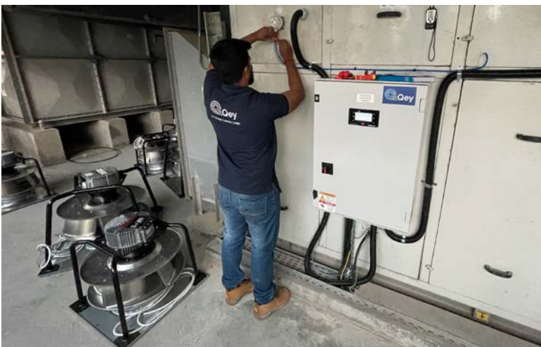
FIGURE 2: Instead of a single fan, FanGrids were installed in the four AHUs. The pre-prepared fan pack-age makes installation quick and easy.
