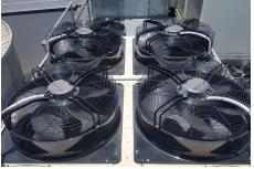
ebm-papst monitored a condenser with 5 fans, for medium temperature rack, with compressor 1 on a VSD and compressor 2 and 3 with a soft starter to measure and verify the avoided energy use.
